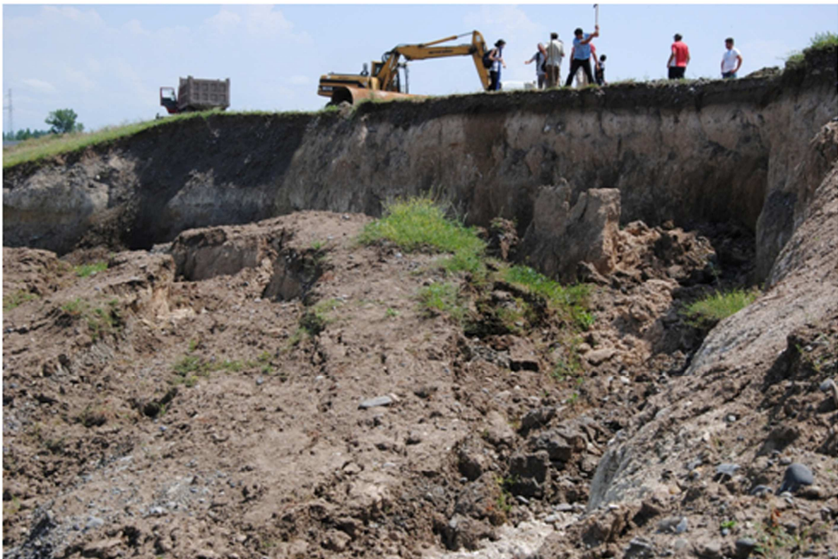
Fig. 21. Doghlauri cemetery, view of the damaged area, from W.
